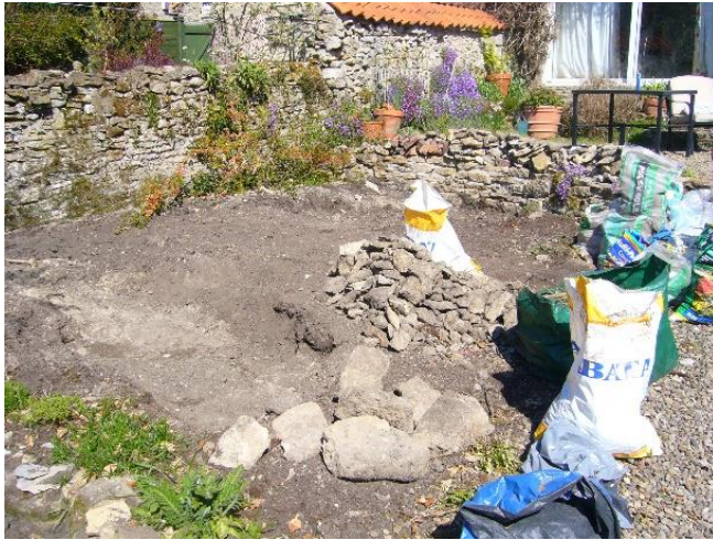
Fig2: Digging out the rocks.
